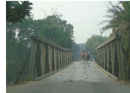
Narrow bridge in Sultanpur to ALC station
