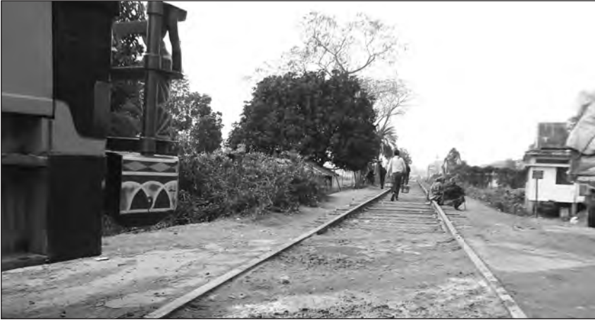
Picture 5: Poor Condition of the Rail Line Passing through Connecting Roads
