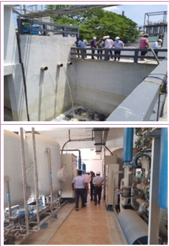
Source: Field visit to India
