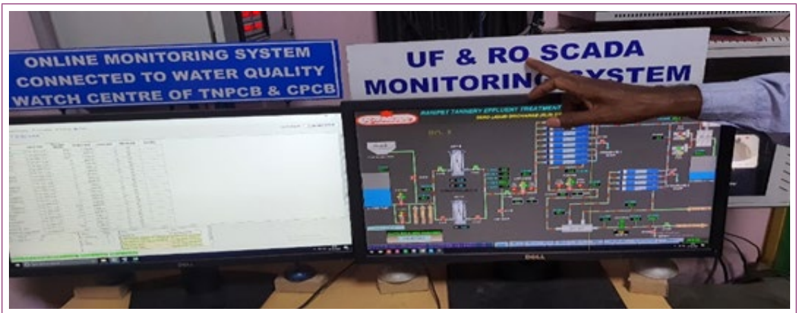
Source: Field visit to India
