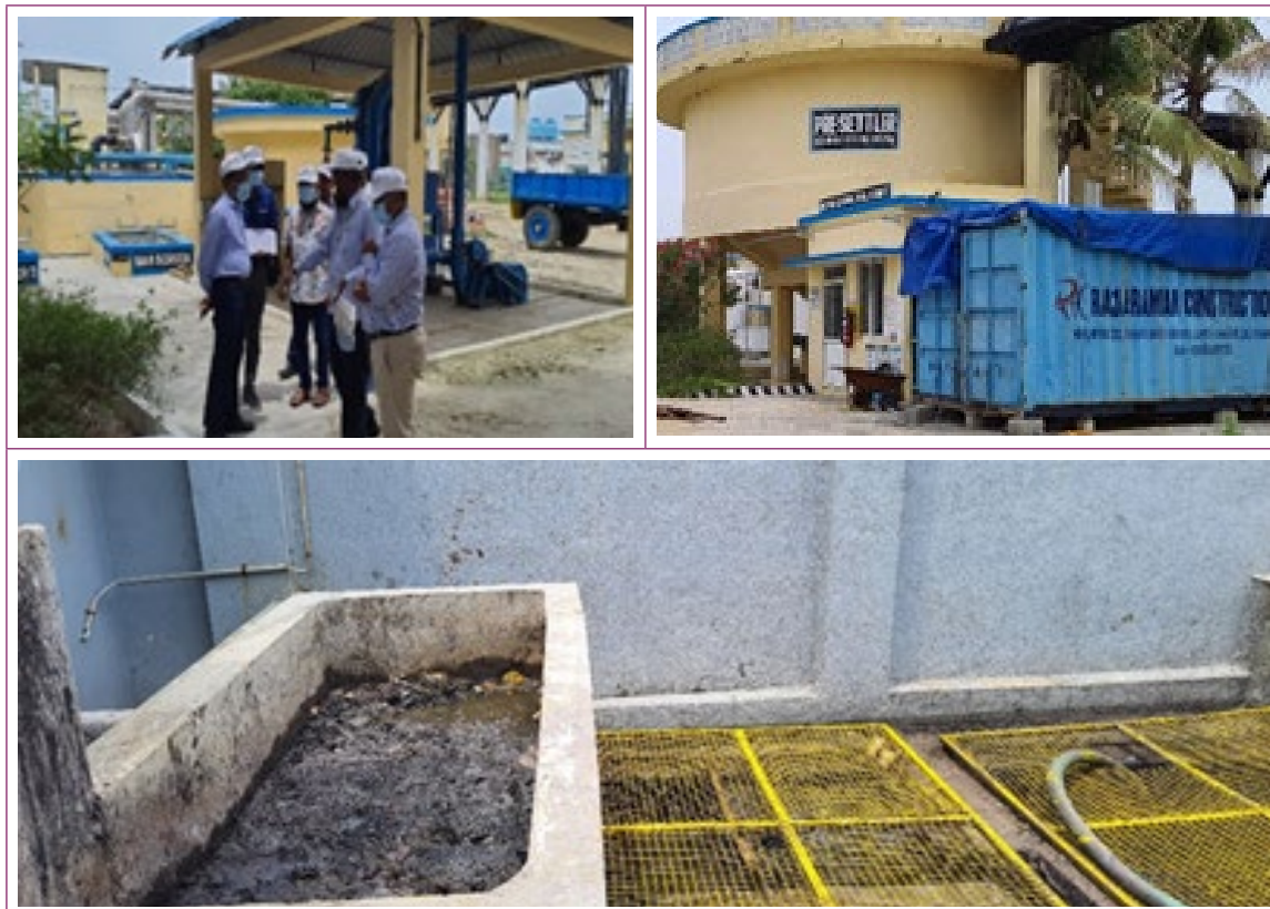
Source: Field visit to India
