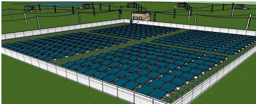
Fig. 3. Solar panel mounting
